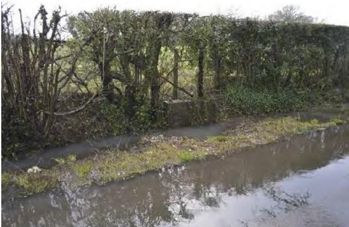
Fig 2: Minor example of flooding as previously observed during FRA site visit
