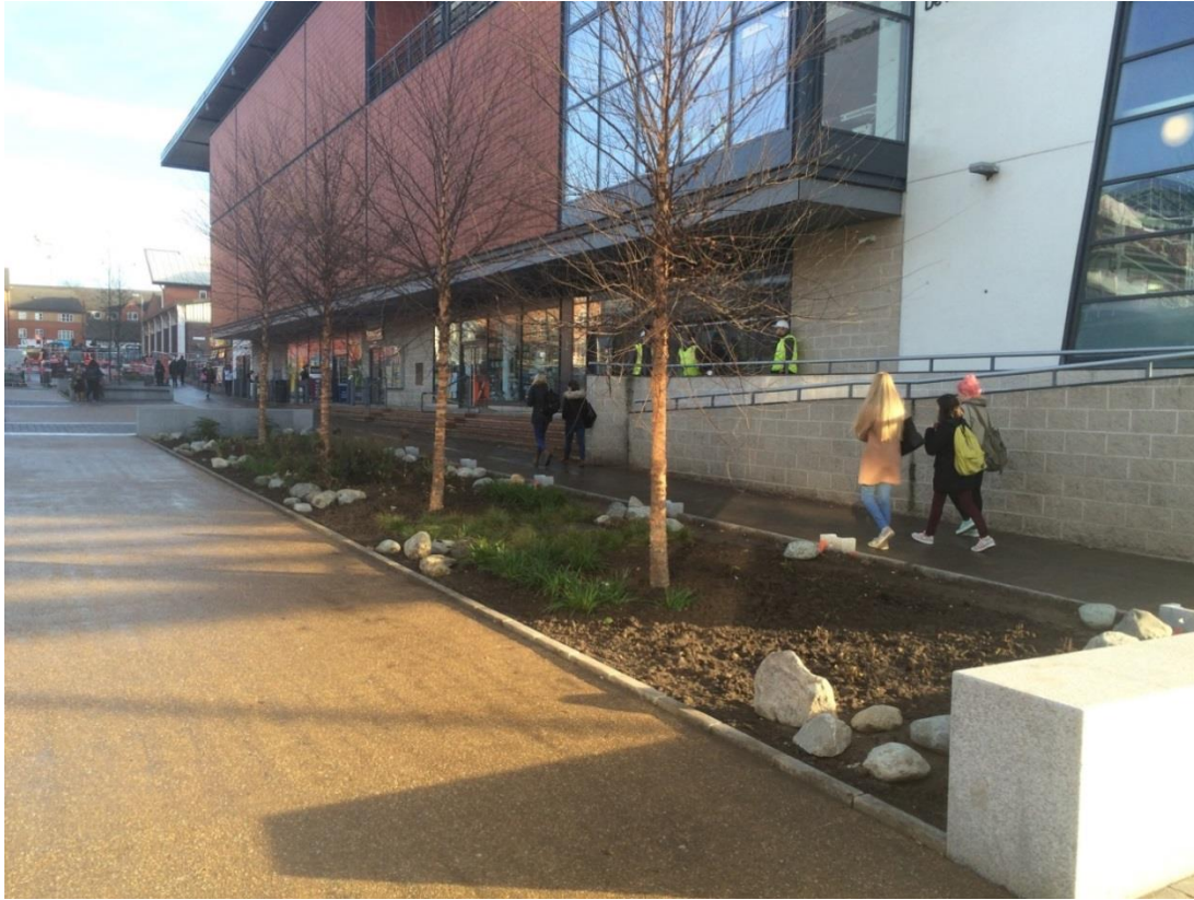
Fig 4: Nearing completion December 2015
