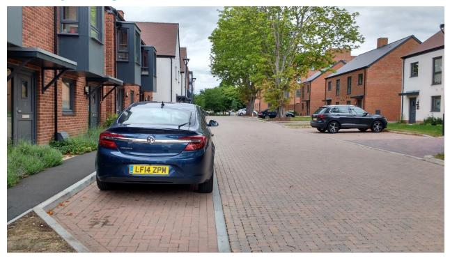
Fig 1: Permeable Paving within Parcels. Waterbutts on each house to the rear.
