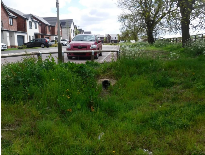
May 2020 showing swale and outlet from piped section close to trees
