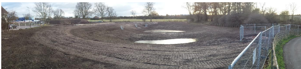
Pond under construction winter 2017
