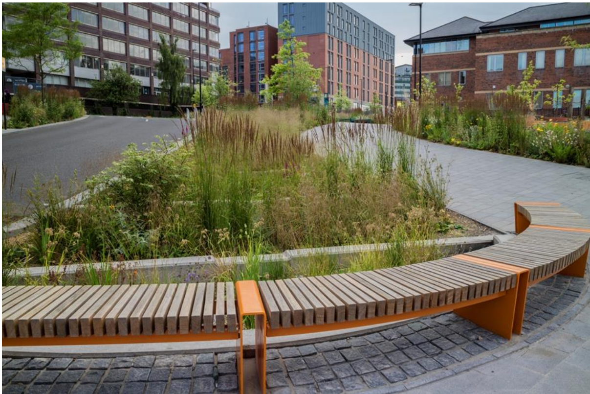
Fig. 2 SuDS cascade through areas of significant level change, together with wetland planting – Photo SCC
