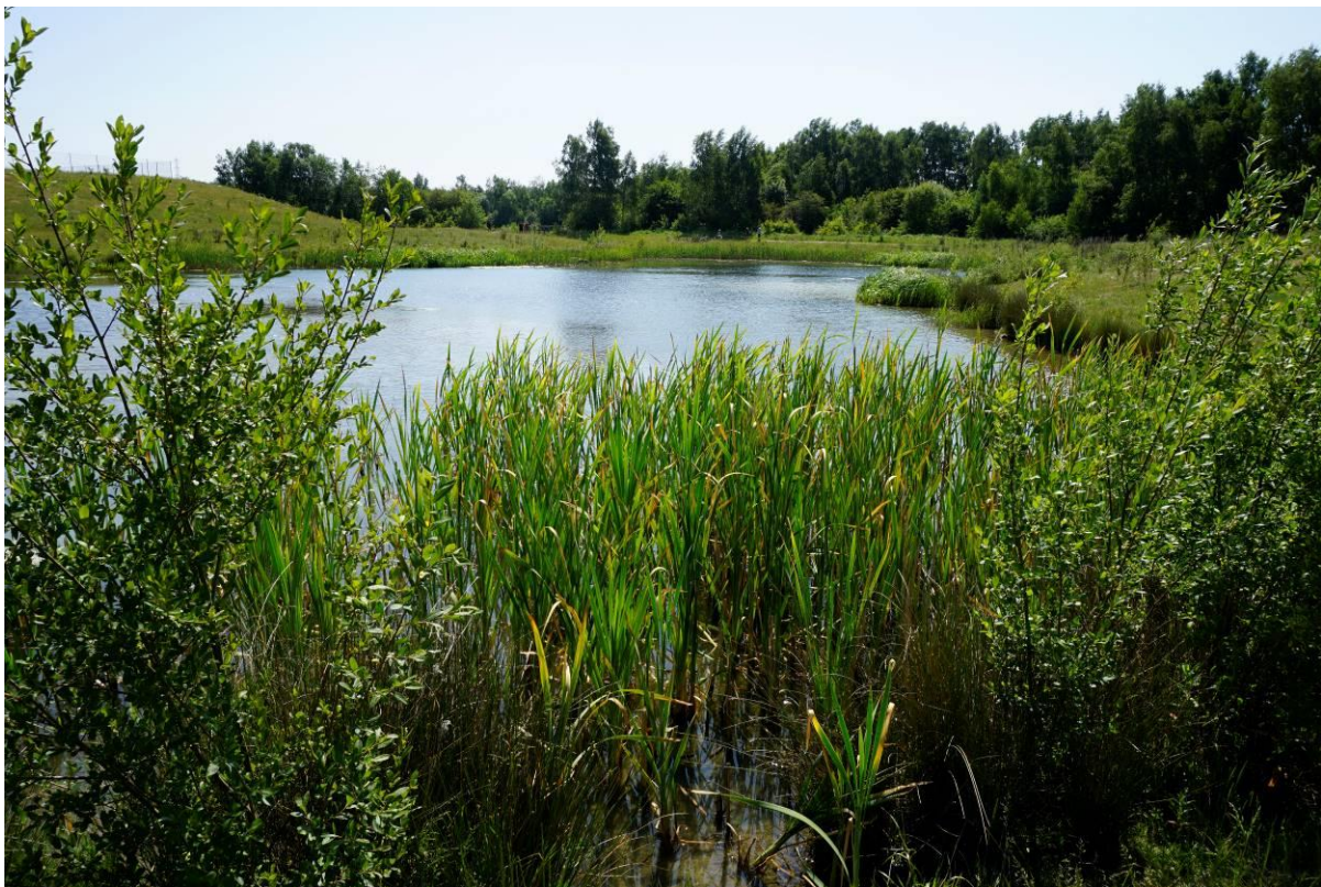
Fig 1 the largest pond in the Markham Vale North SuDs, designed to have permanent open water as well has storage capacity for a 100 + 30% flood event.
