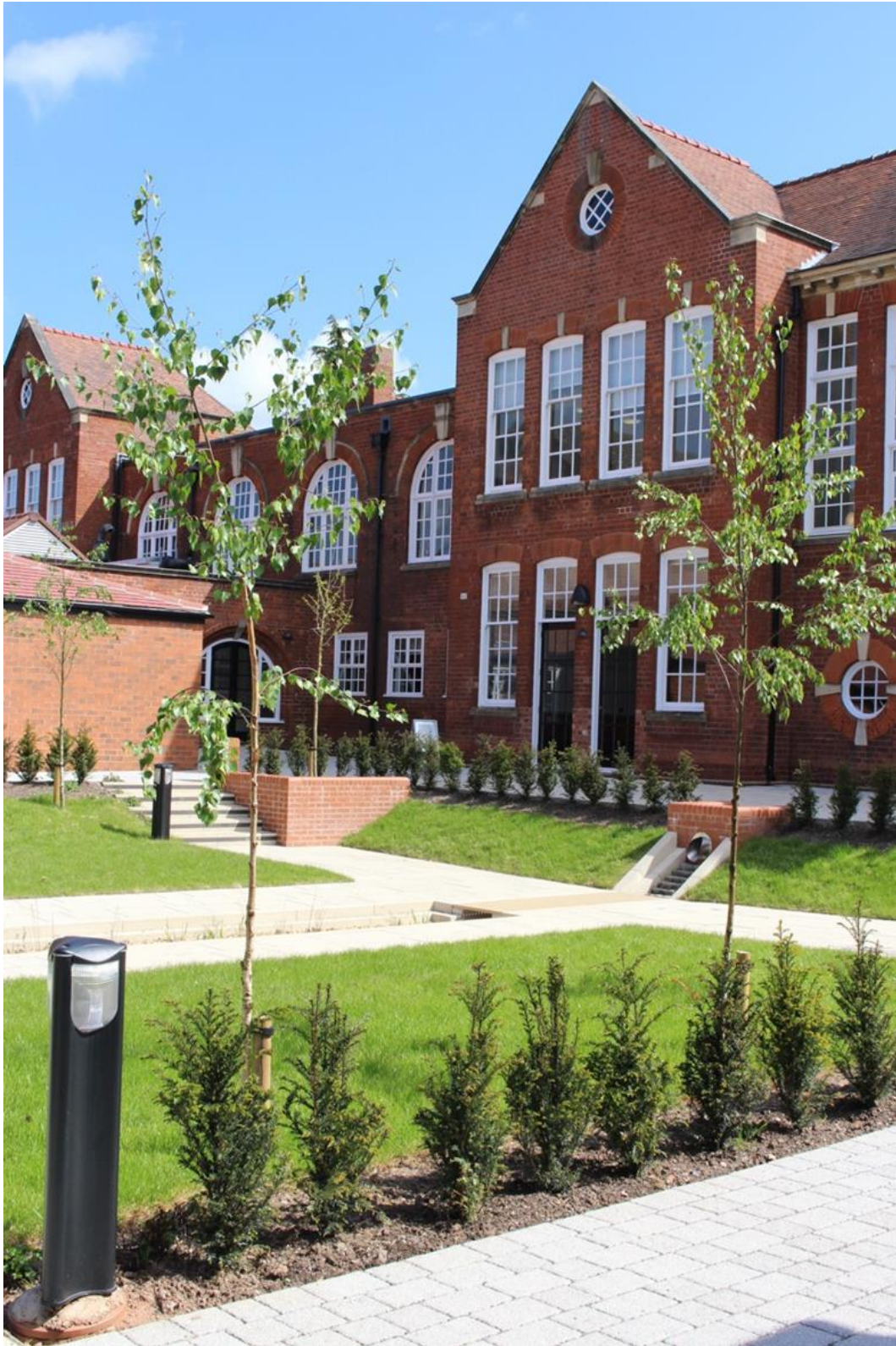
Fig 1: School building and SuDS court
