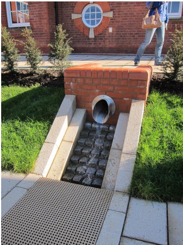
Fig 5: Solar powered water spout
