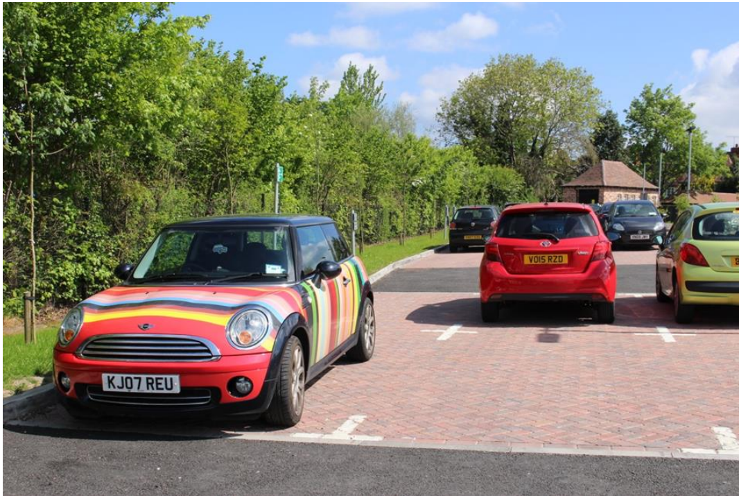
Fig4 : Permeable block paving to car park
