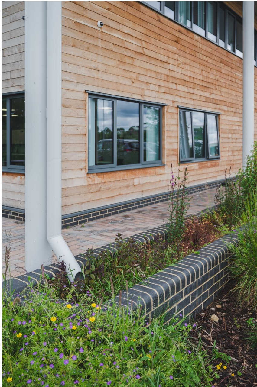
Raised wetland feature and one of a number of rainwater pipe inlets.
