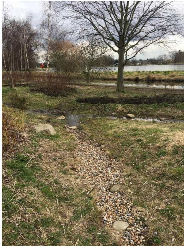
Fig 3 – Surface water collected in an infiltration trench following a storm event, next to the New River and West Reservoir
