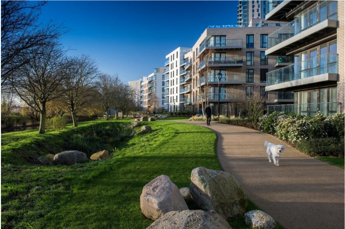
Fig 2 – Play/seating boulders integrate the partially planted swale as a multifunctional landscaping feature, bordered by newly planted trees and a permeable path.
