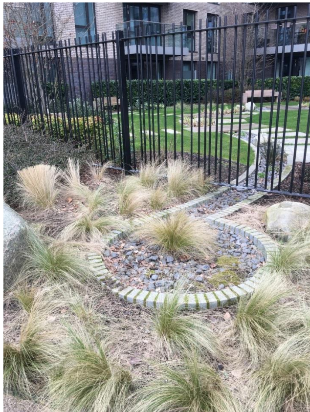
Fig 5 – Example of how SuDS have been used to link areas of the scheme and give character.
