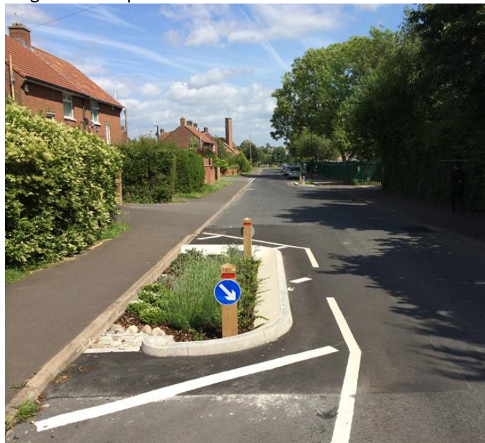
Fig 6: New rain gardens on Embleton Road
