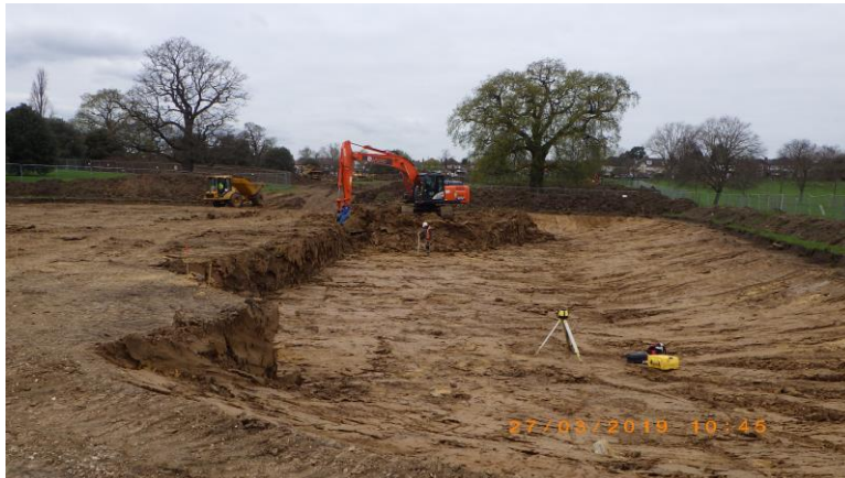
Initial excavation of clay (late March 2019)
