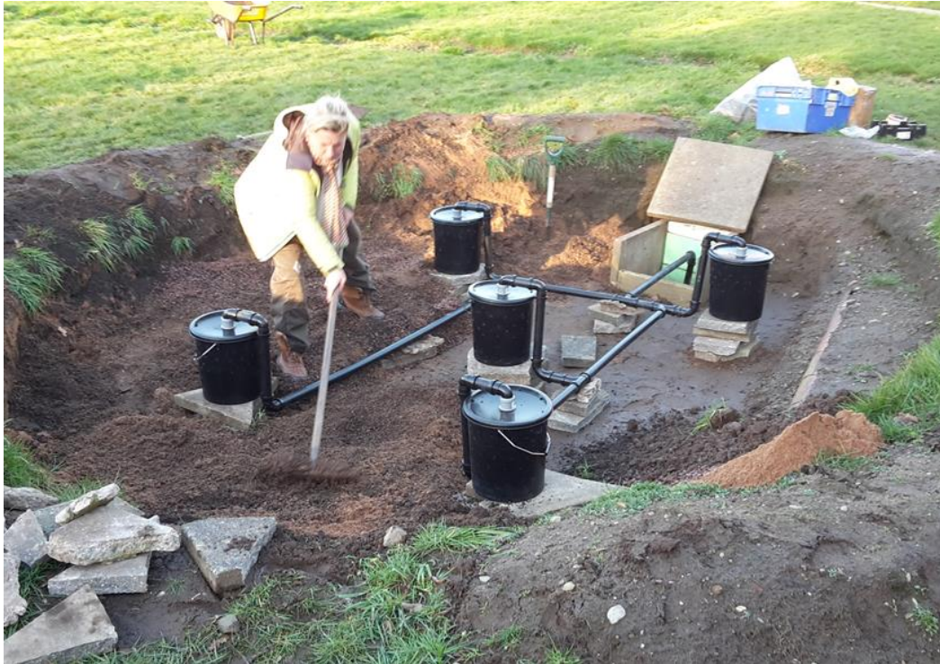
6. Testing silt-trap buckets being for water-flow
