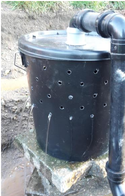
7. Grozone volunteers wrap buckets with geotextile and complete rain garden back-fill
