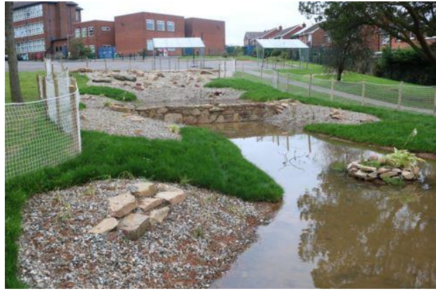
Fig. 3- Detention ponds with intermediate cascade.
