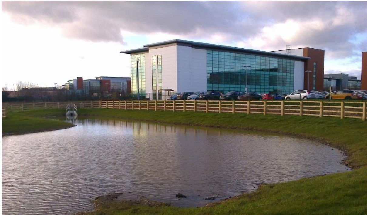
Fig1 Surface water retention pond at Longbenton High School
