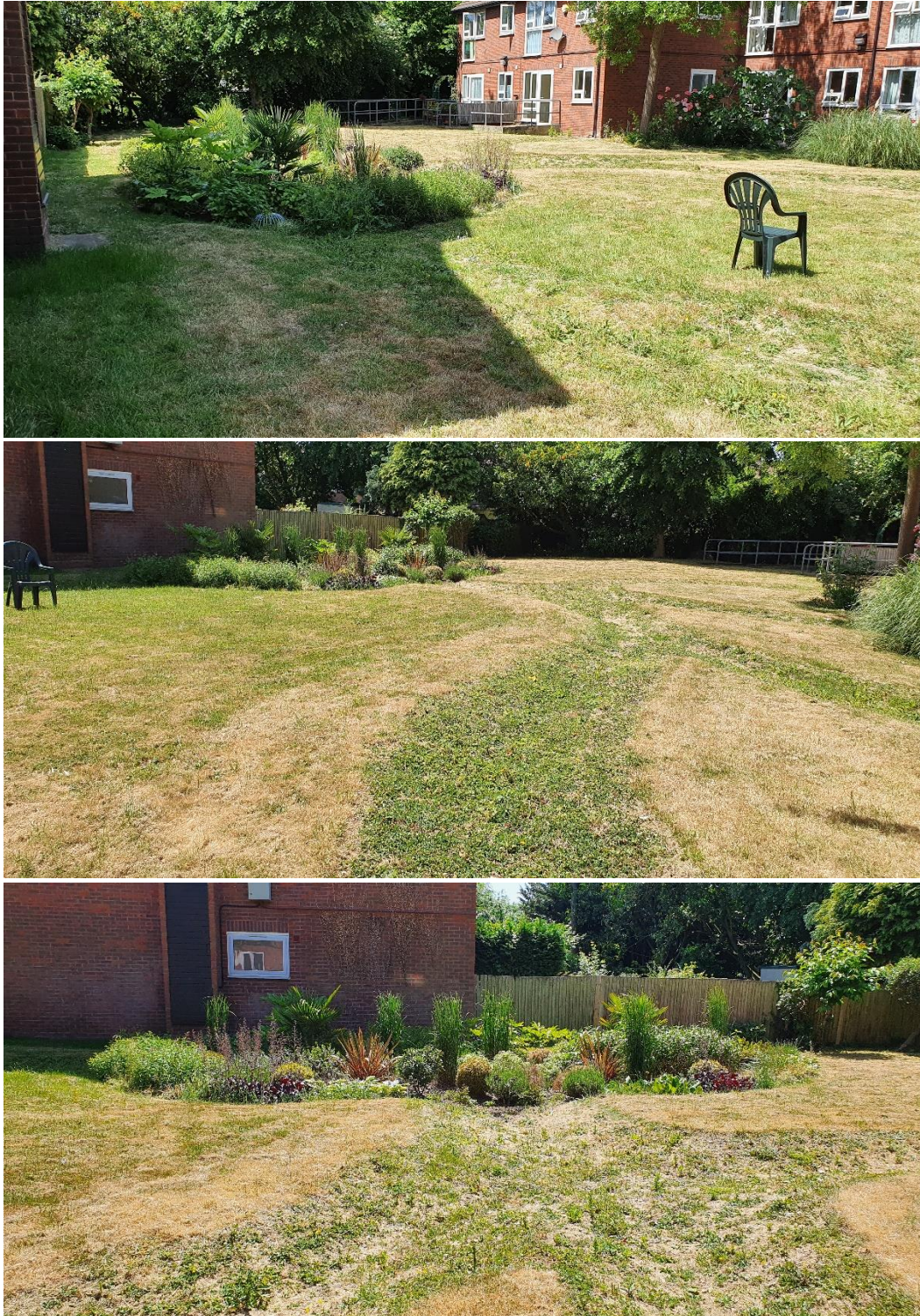
Phase 1 swales and rain garden
