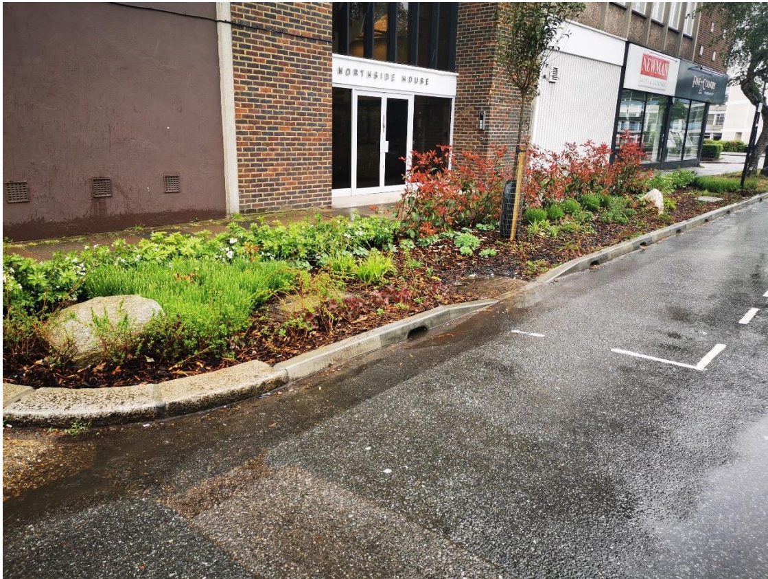
Phase 3 roadside rain gardens and wildflower turf
