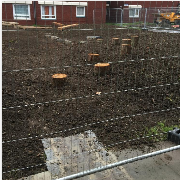
Fig. 6: During the construction of Play logs and Boulders
