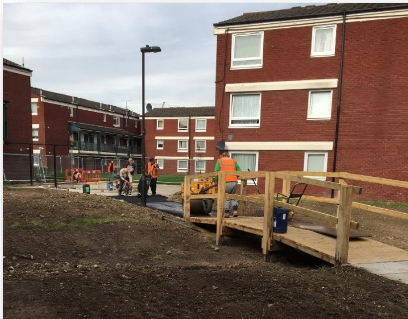
Fig. 5: During the construction of wooden Bridge and East side of scheme
