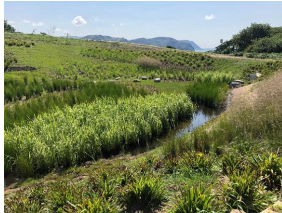
Figure 3 Photo on completion
