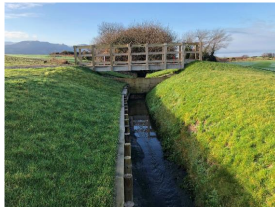
Figure 5 Timber weir and footbridge
