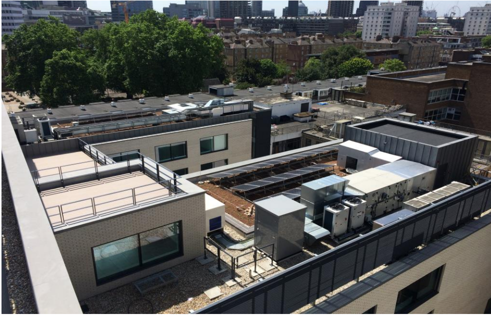
Roof zone 15 with the biodiverse area visible surrounding the PV panels
