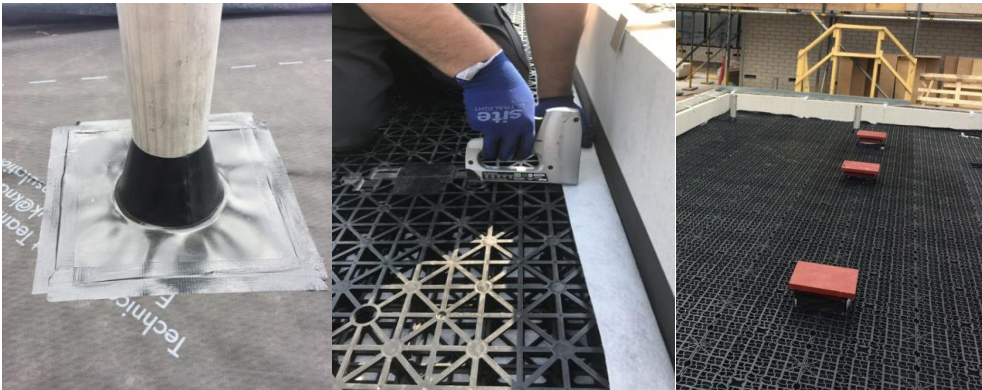
Penetration detail around man safe post
