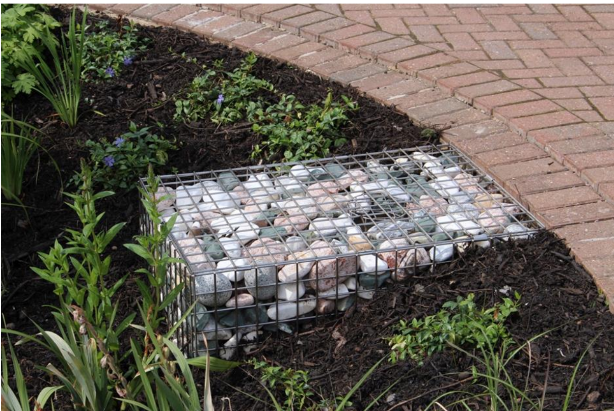
Fig 6: Raingarden Outlet Basket, Year 1
