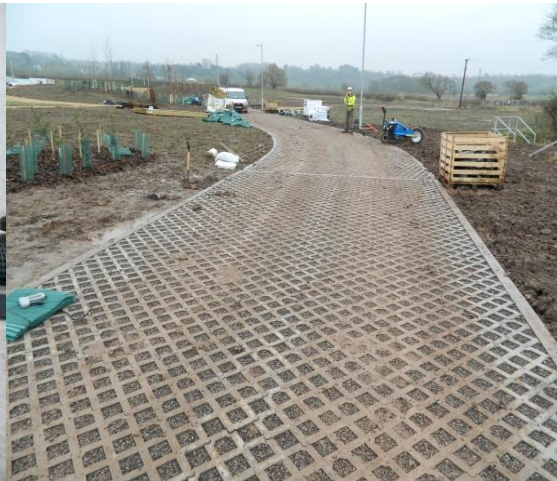
A section of the permeable paving access road
