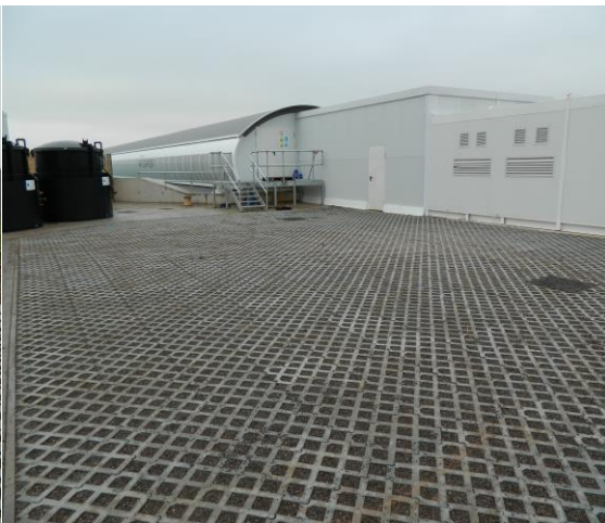
Maintenance yard area
