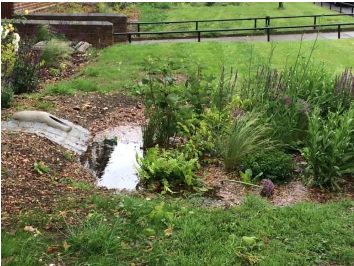
Fig 7: The rain gardens successfully storing water in a heavy rainfall event
