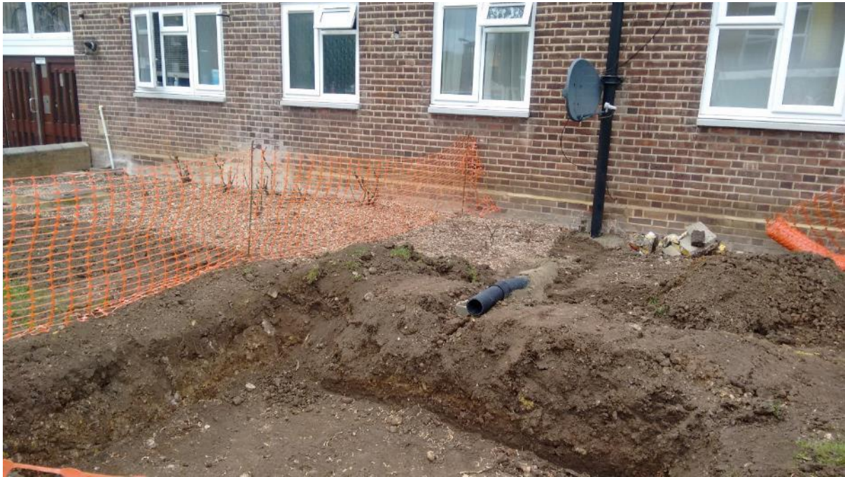
Fig 4: The gardens during construction, with overflow pipe
