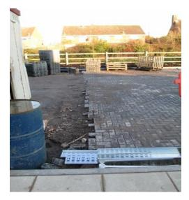
Figure 7 Porous paving was used for the main car park areas
