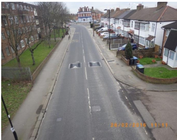
Figure 1 Alma Road before
