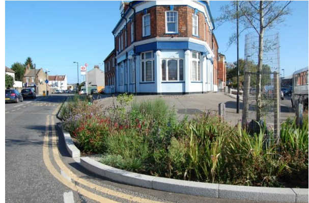
Figure 4 Alma Road/Scotland Green Road junction after with permeable footway
