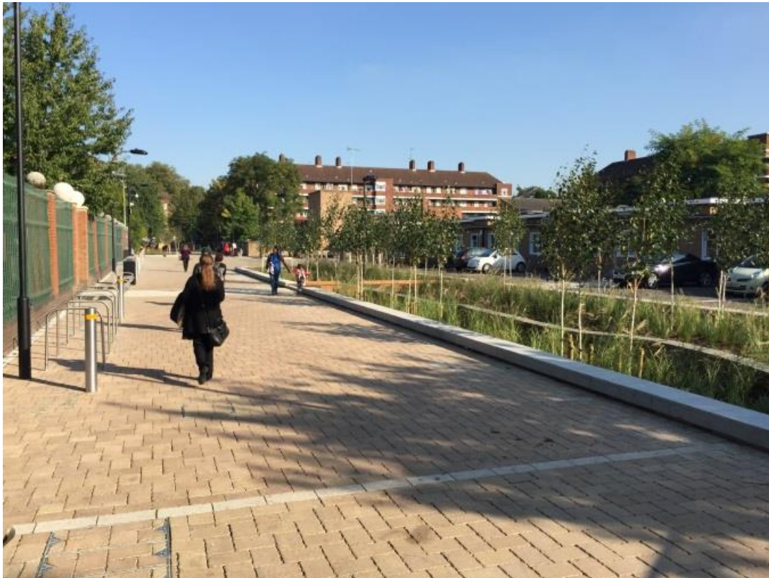
Figure 5 Permeable paving directs water to heavily planted basins
