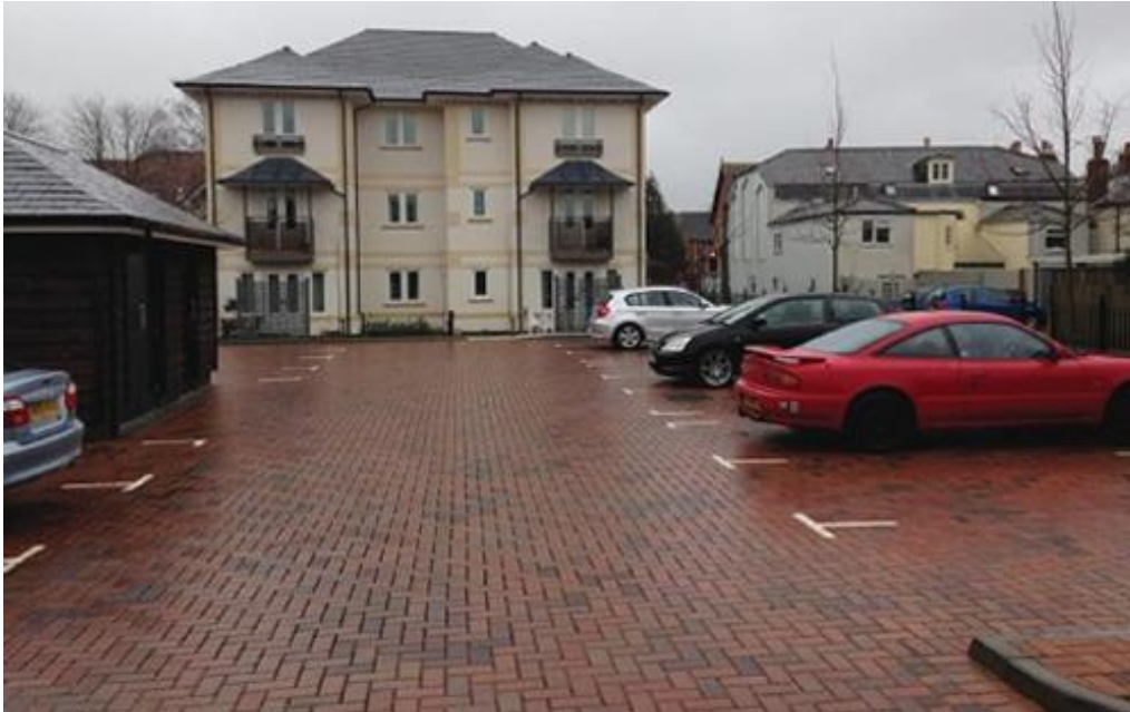
Figure 5 Buckland House Car Park (3)
