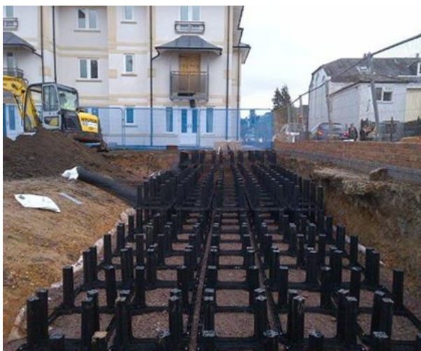
Figure 3 Buckland House Car Park construction phase (1)
