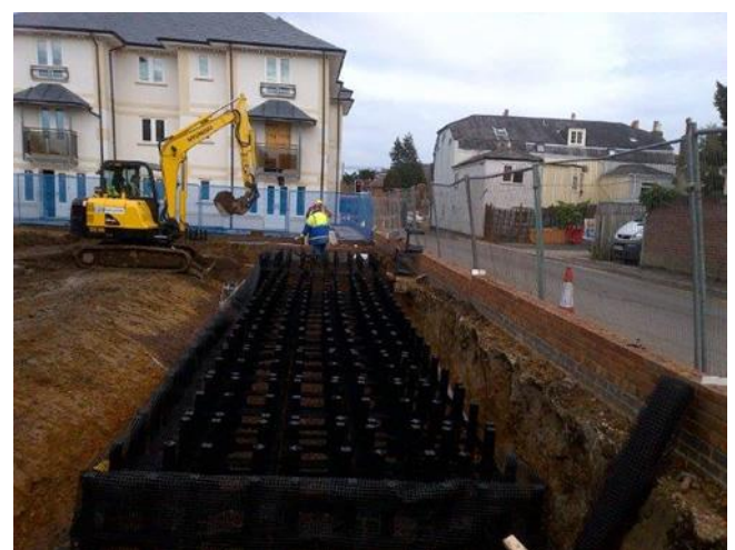
Figure 4 Buckland House Car Park construction phase (2)
