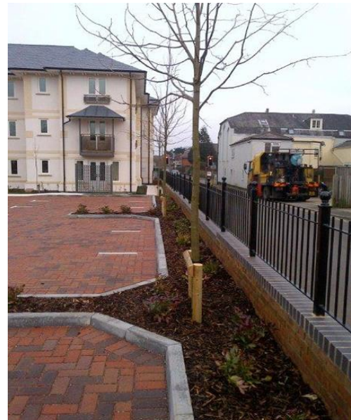
Figure 2 Buckland House Car Park (2)
