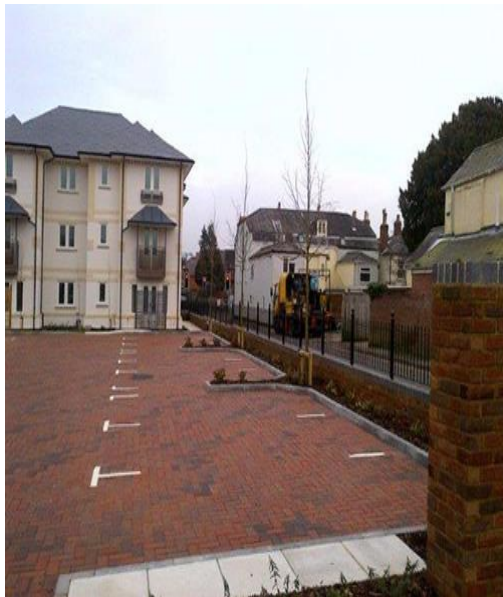
Figure 1 Buckland House Car Park (1)
