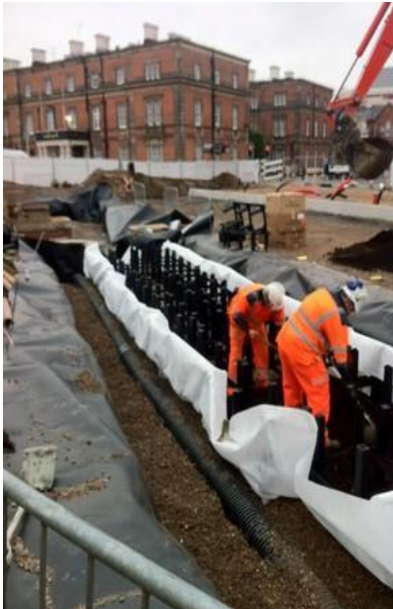
Figure 2 Construction of tree pit
