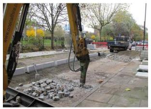
Figure 12 Original road bed revealed for rain garden and pipe connection routes to be created
