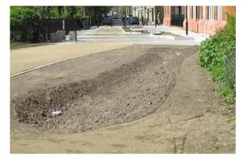
Figure 13 The swale formed
