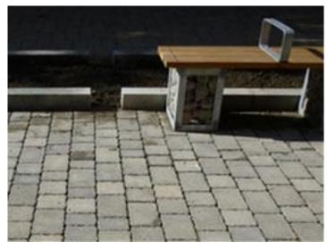
Figure 7 Permeable block paving
