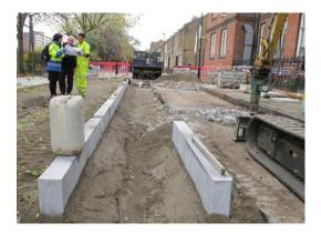
Figure 14 Lining up the rain gardens. Working back from the lowest point to attain enough fall, November 2013
