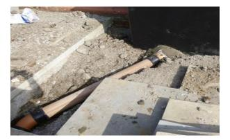
Water is collected from the roof of Oxford House in the attenuating rainwater planters, when at saturation point an overflow point discharges excess water under the footway and permeable paving and into the rain garden, shown in Figure 14.
