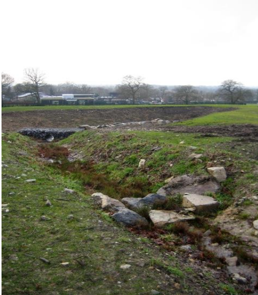
Figure 1 SuDS basin under construction
