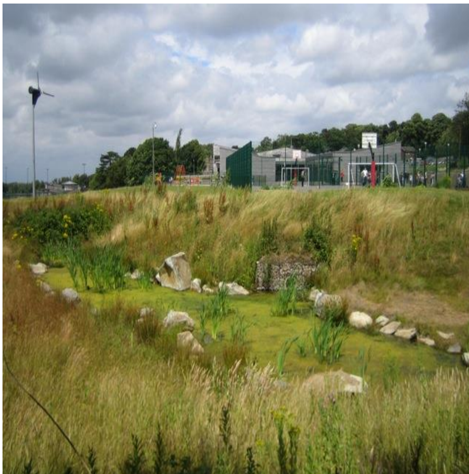
Figure 7 Completed basin (July 2010)
