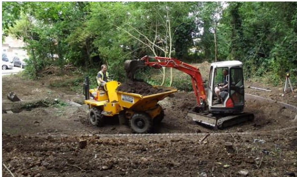
Figure 2 Construction of wetland
