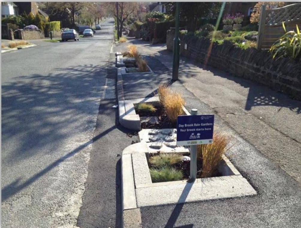
Figure 5 Completed rain gardens (1)
