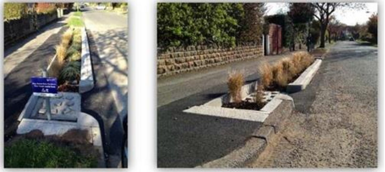
Figure 6 Completed rain gardens (2)
