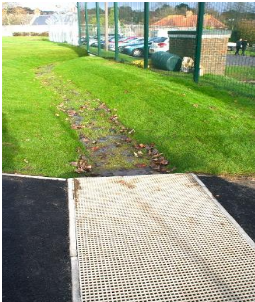
Figure 1 Bridge construction (before swale planting) allows shallow swale depth and grating surface intercepts path runoff
