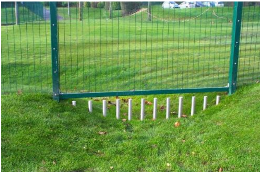
Figure 2 Stainless steel pins provide security at the site's secure boundary
