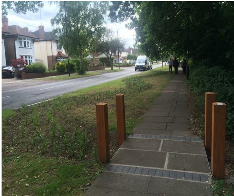
Figure 5 Completed swale
