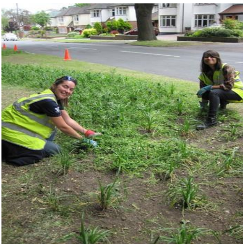
Figure 3 Volunteers weeding the swale
