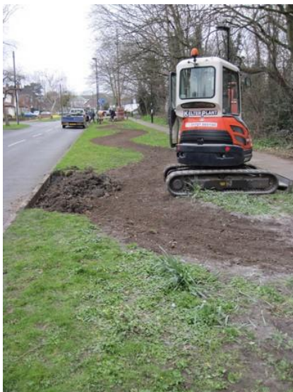
Figure 1 Constructing the swales
