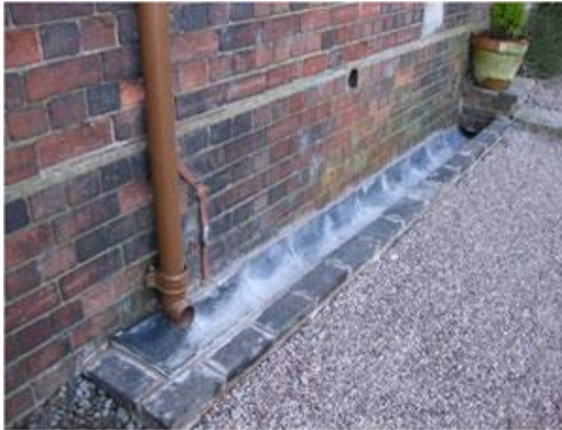
Figure 3 Completed build around the existing downpipe
