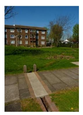
Figure 2 Ornamental rain garden (early after installation) showing a channel bridge under a pathway
