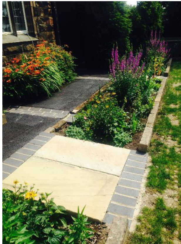
Figure 3 Brick rain channel and linear raingarden in front of the old caretaker's house (2)
