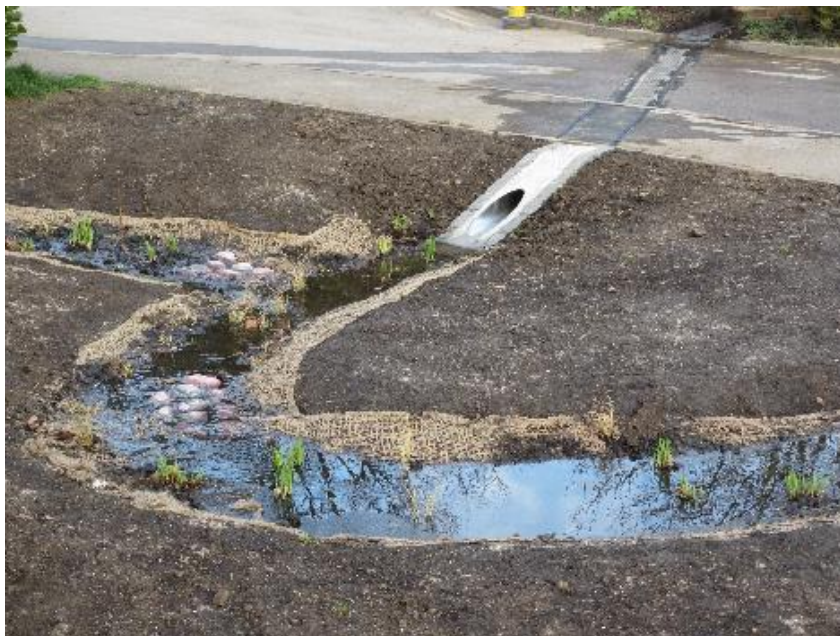
Figure 6 Inlet from what the community described as 'raincatcher' grating across the access road
