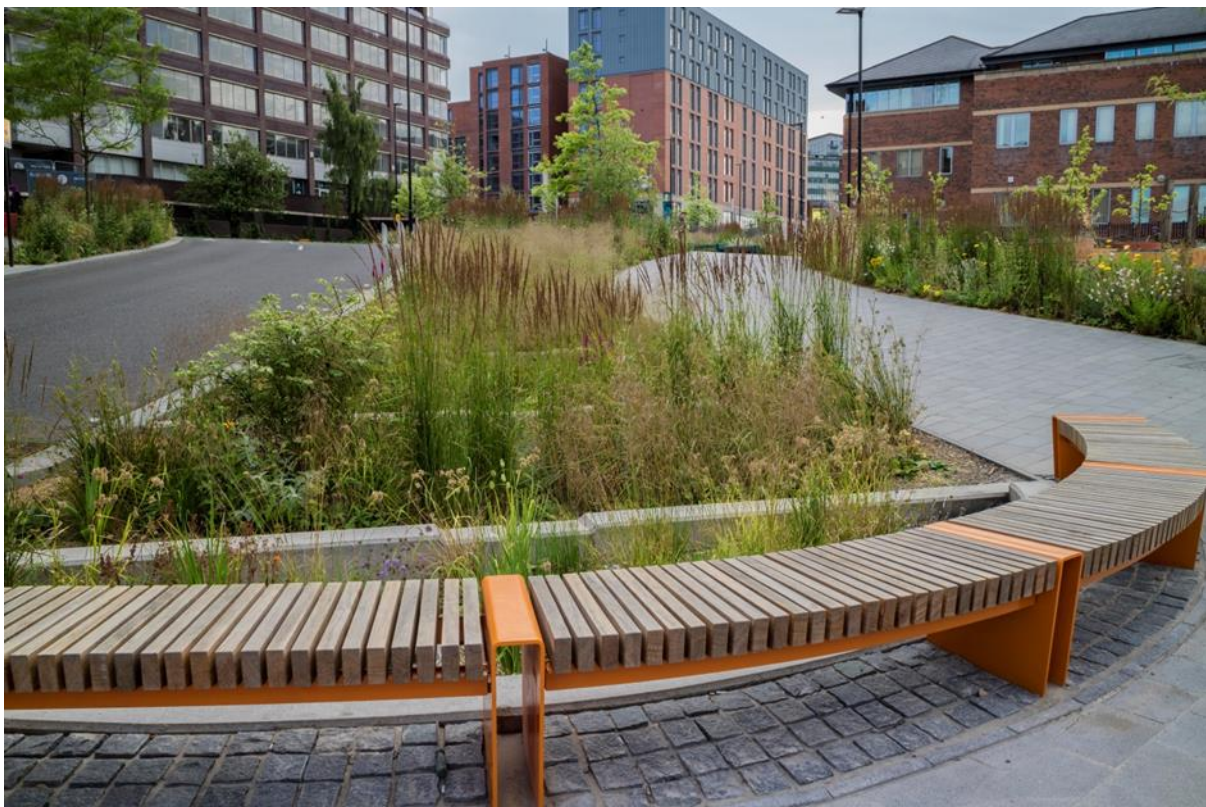
Fig. 2 Suds cascade through significant areas of level change, together with wetland planting – Photo SCC
