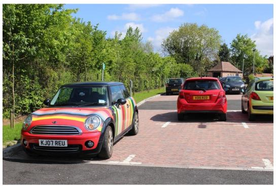
Fig4 : Permeable block paving to car park
