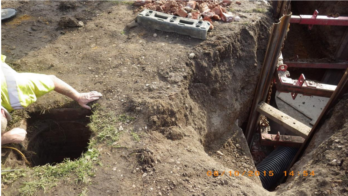
Figure 4 Constructing a new outfall
