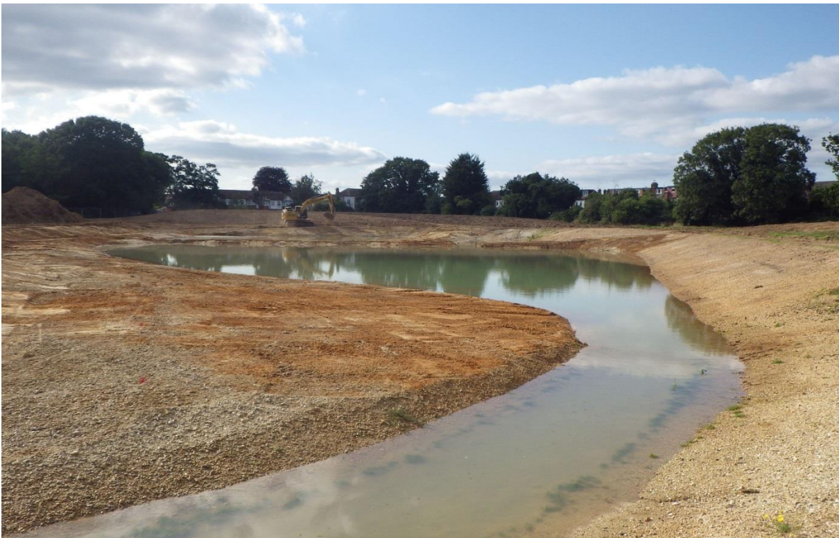
Figure 3 Construction of wetland cells
