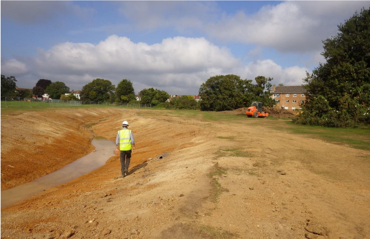
Figure 2 Firs Farm Site after completion of Phase 1
