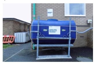
Figure 3 Rainwater harvesting tank at Cramlington Treatment Works
