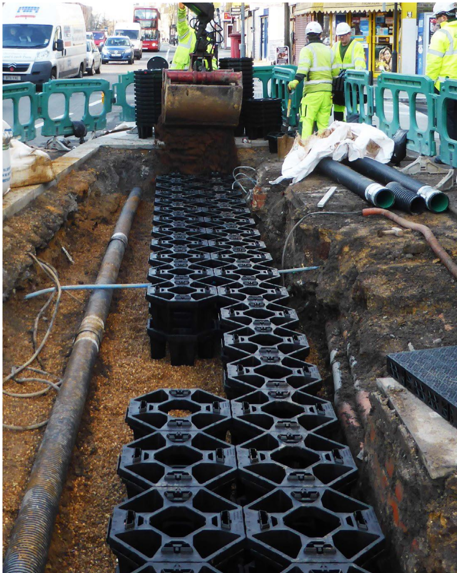
Fig 3: Tree pit cells being filled during construction
