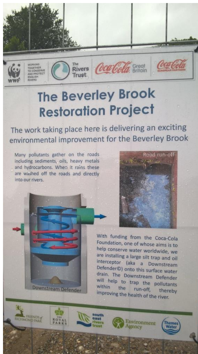
Fig 1: Public Information Sign during construction
