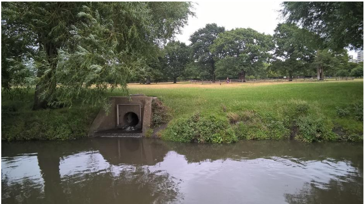
Fig 3: Existing Outfall to Beverley Brook
