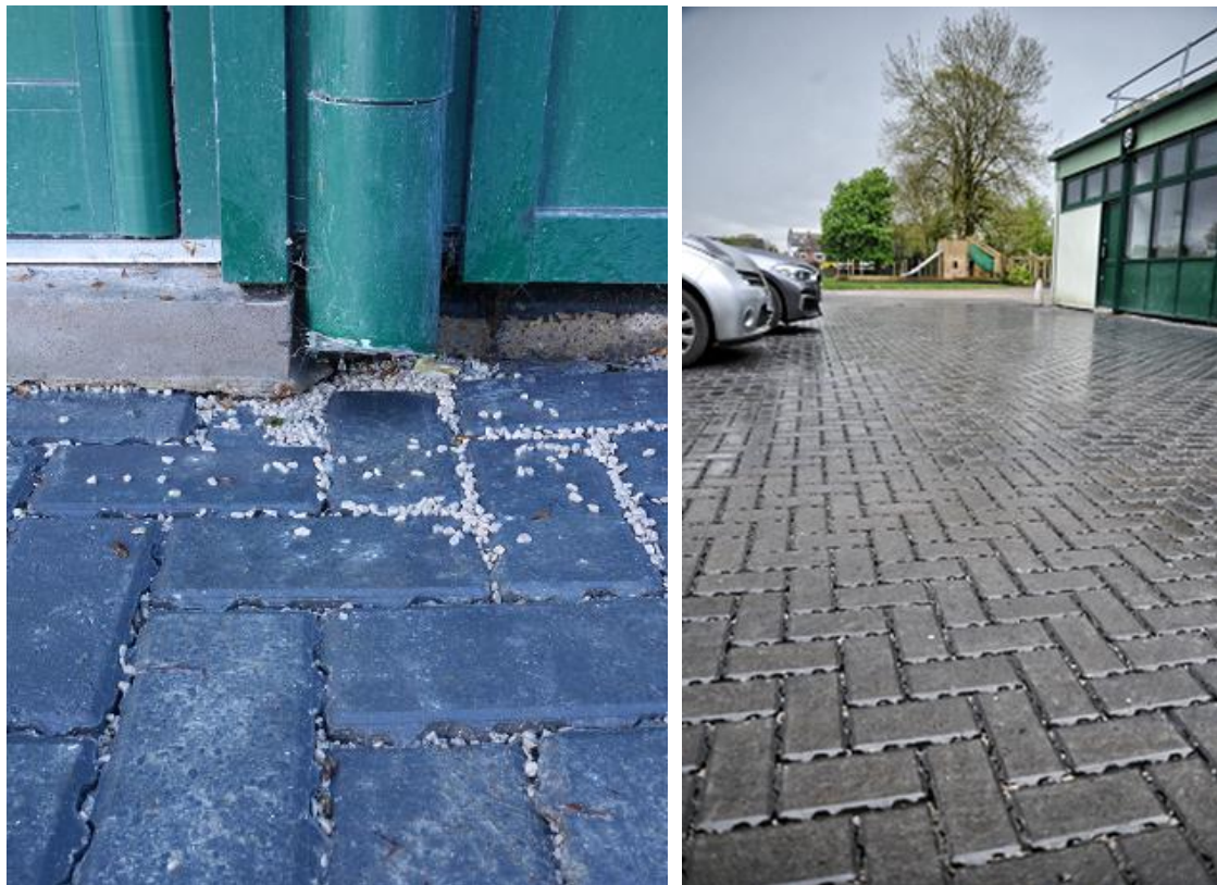
Fig 5: Permeable paving replaces an existing tarmac car park and offers a SuDS solution where space is at a premium
