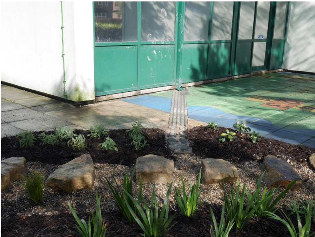
Fig 3: Fluted drain and river washed cobble cascade transfer surface water to the raingardens
