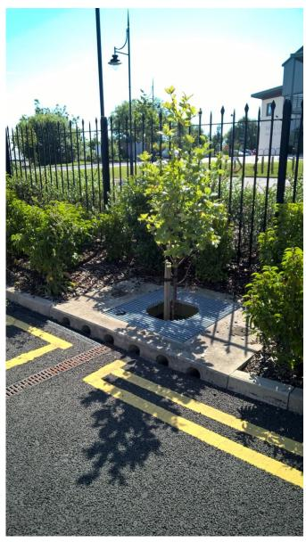
Fig 1: Biofilter unit with combined kerb inlet and channel drain inlet
