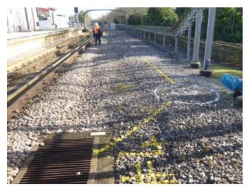
Fig 2: Setting out works
