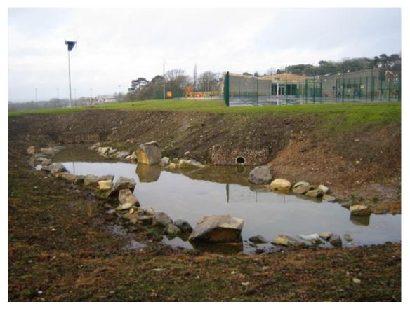
Fig 3: SuDS shortly after construction and un-vegetated
