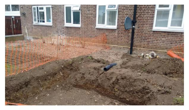
Fig 4: The gardens during construction, with overflow pipe
