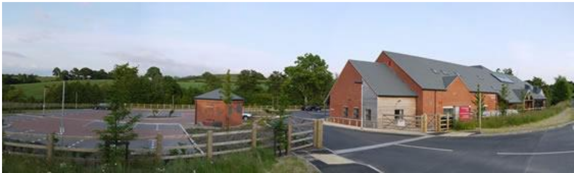
Figure 1 Kington Medical Centre entrance
