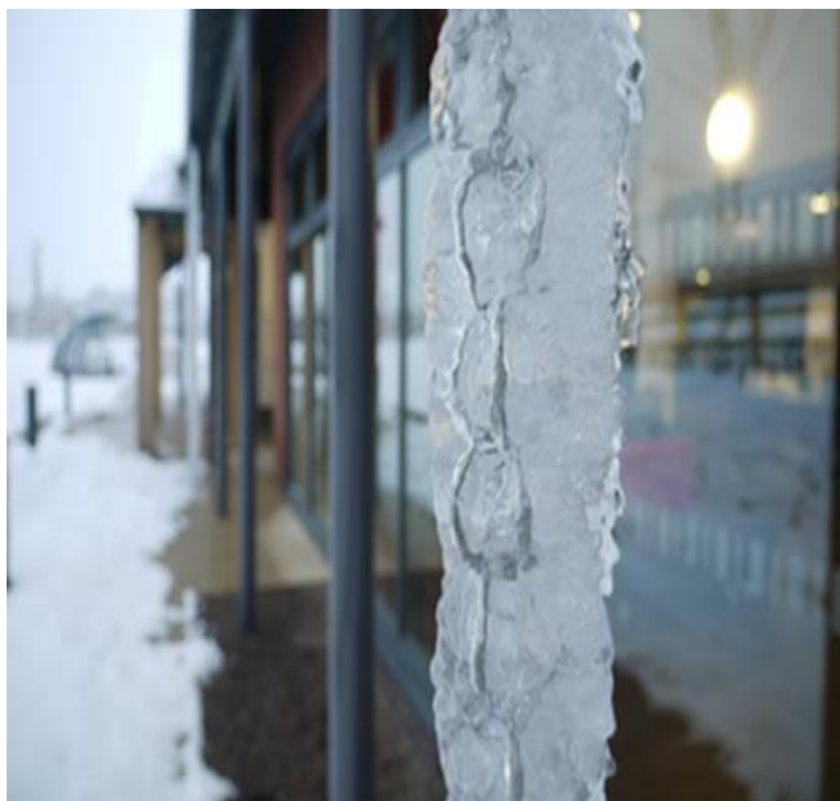
Figure 9 Rain chains were used by the architects to create an interesting feature using rainwater runoff
