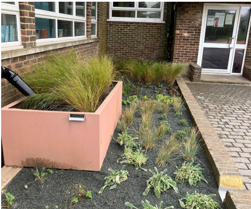
Figure 8: Large rain planter and rain garden
