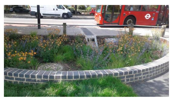
Fig. 2: Established Rain garden - Collecting surface water during storm event
