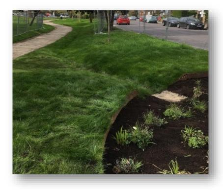
Fig. 6: After the Construction and linked with swale and other SuDS.
