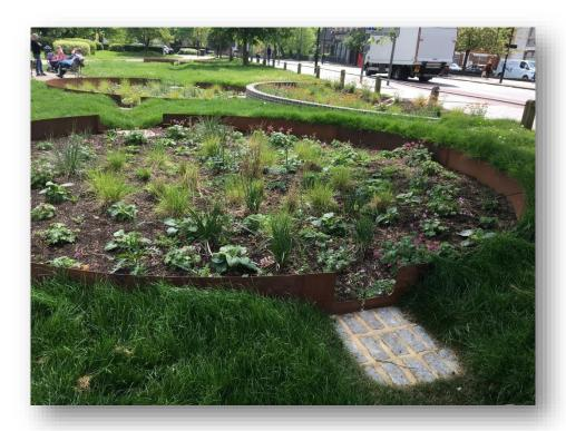
Fig. 3: Example of SuDS and Management Train used to link the areas and give character to the scheme. Also attracting people to interact with SuDS features.
