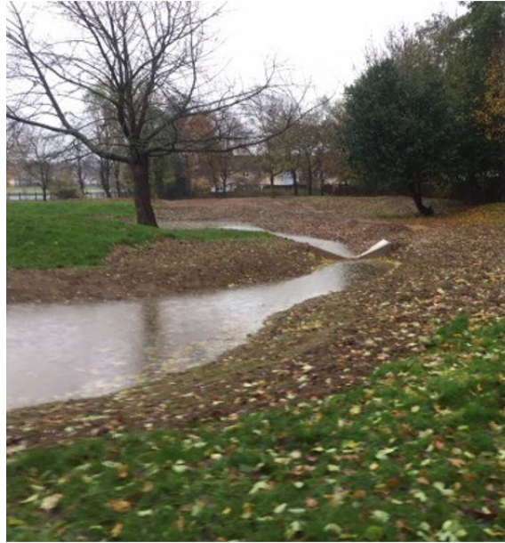
Fig. 6 – The upper basin reducing storm water runoff during storm Angus.
