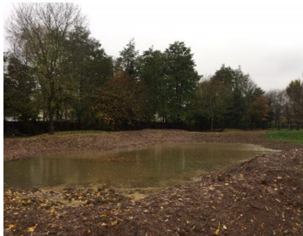
Fig. 7 – The lower basin reducing storm water runoff during storm Angus.
