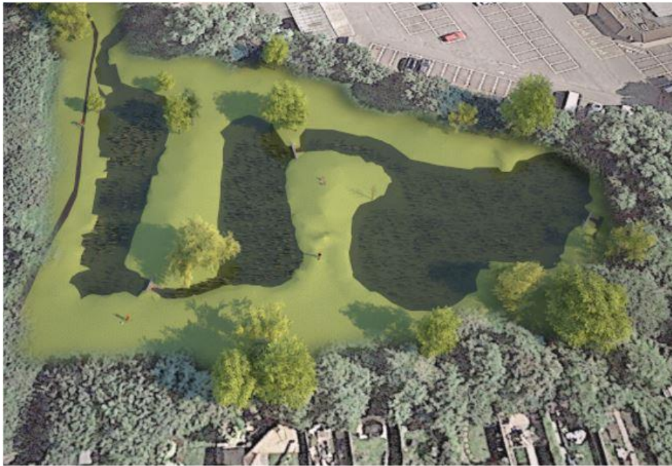
Fig. 2 – This remarkably versatile SuDS scheme is designed to convey runoff water during extreme weather conditions.
